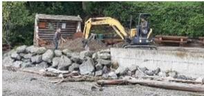
The picnic area bulkhead had some pretty extensive repair work done. The wall is about one foot higher and the area behind the rocks has been engineered so the erosion problems should be alleviated. Dave Heron and
